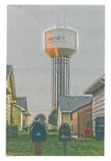
Water- The City of Cheney built a 400,000 gallon water tower in 1992 to address current and future growth and water needs. Three wells supply the City water, which can produce water for up to 4,000 citizens based on 100 gallon per capita per day. 80% of the water infrastructure was replaced in 1974. Water mains from 1919 were replaced in 2008. Typically water mains are designed to last 50-60 years, which means water main replacement could begin in
